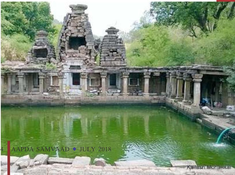
Ramtek Model - Named after the water harvesting structures in Ramtek, Maharashtra. An intricate network of groundwater and surface water bodies, this system consists of tanks forming a chain from the foothills to the plains. Once the tanks located in the hills are filled to capacity, the water flows down to fill successive tanks, generally ending in a small waterhole which stores the residual run-off as well.
